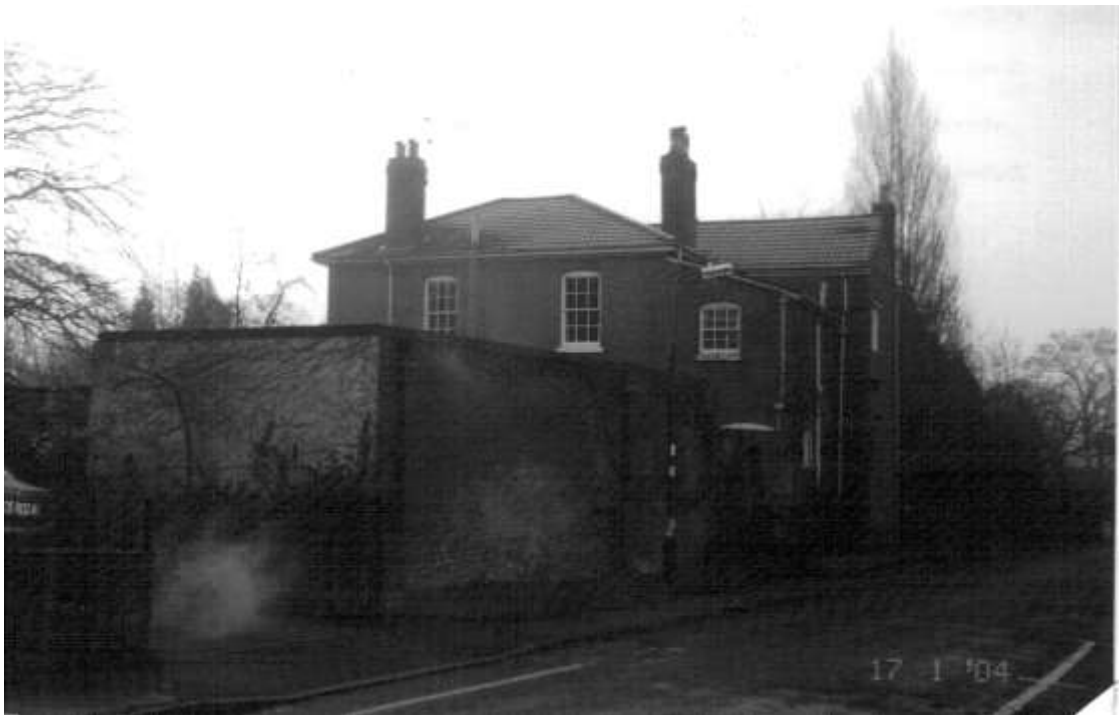
“The Poplars” looking south from Green Lanes; the stable block in the foreground was demolished shortly after this photo, behind is the 1860 extension with the sash windows which were transferred from the ground floor front, and the two-storey lean-to extension of 1900 which was demolished in 2008
