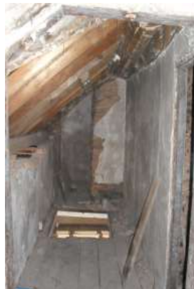
30 High Street, showing the purlins resting on the brick gable and the exposed flues in the wall above the trap door.
