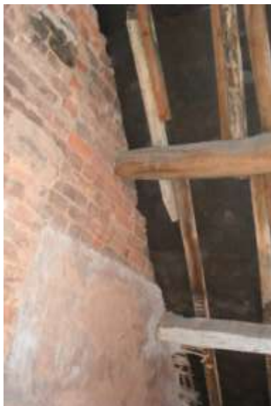
30 High Street, showing the purlins resting on the brick gable and the exposed flues in the wall above the trap door.
