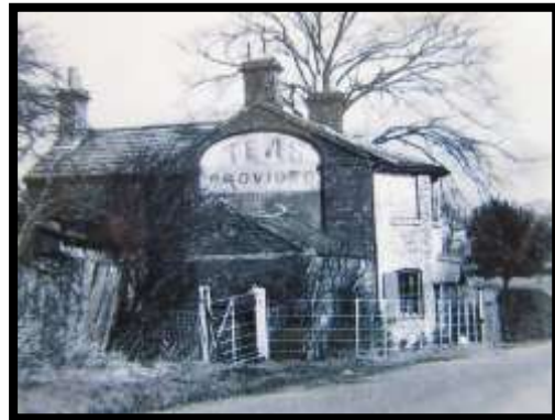
(m) The old Toll House on the Tamworth Road
