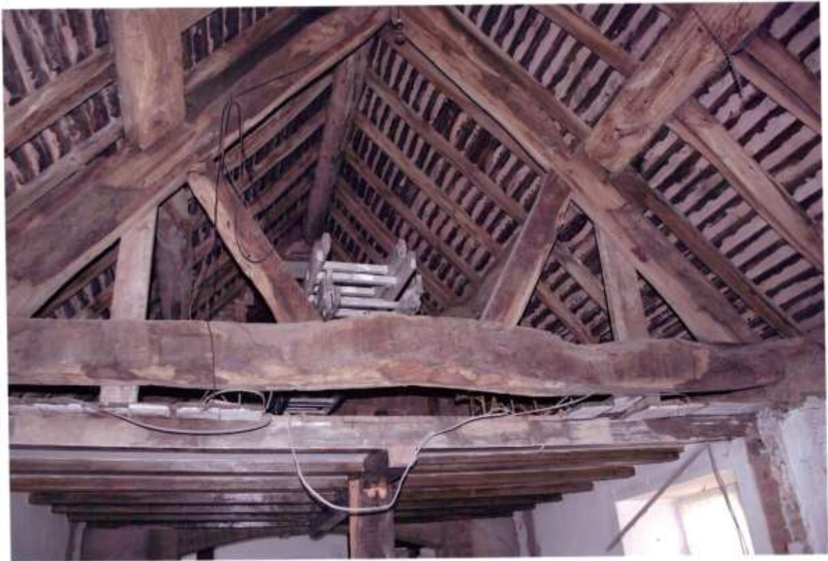
Roof of the rear barn during renovation
