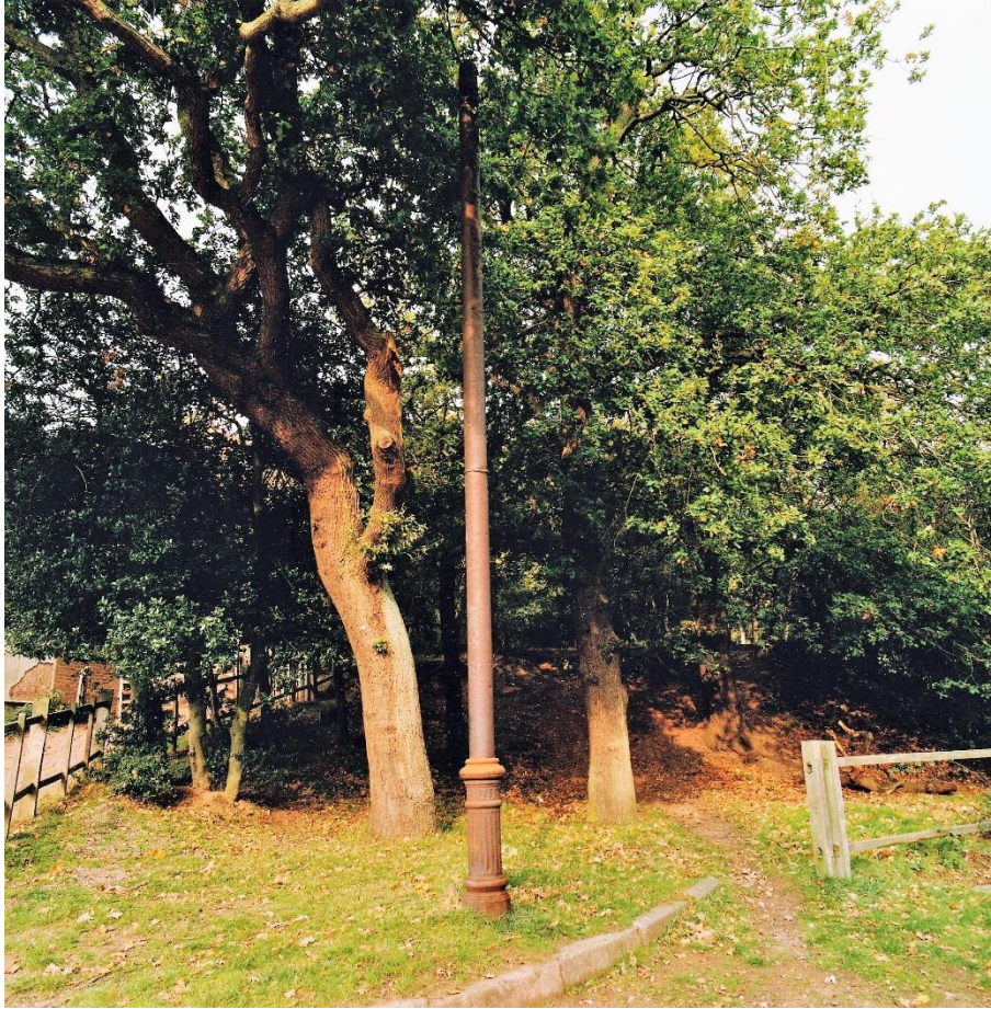
Photo 4 – Stench pipe at the north end of Keeper’s Pool dam, next to the quarry and opposite the old outdoor swimming baths, at O.S. G.R. SP 1073 9656.
