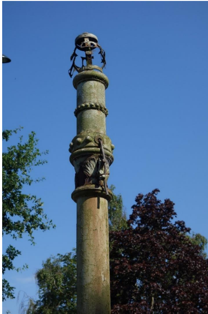
Photo 2 – Details of the vent end of the stench pipe.
