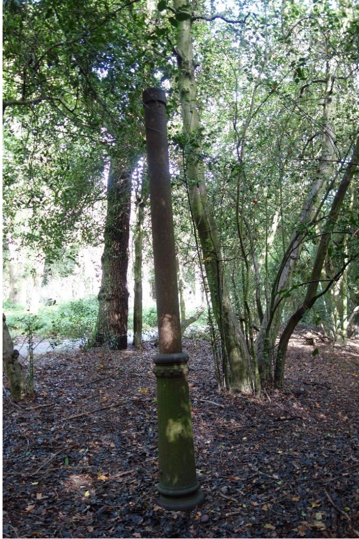
Photo 3 – Stench pipe near Holly Hurst in Sutton Park at O.S. G.R. SP 1073 9572 possibly dating from the First World War. Compare the base of this pipe with that shown in Photo 4.
