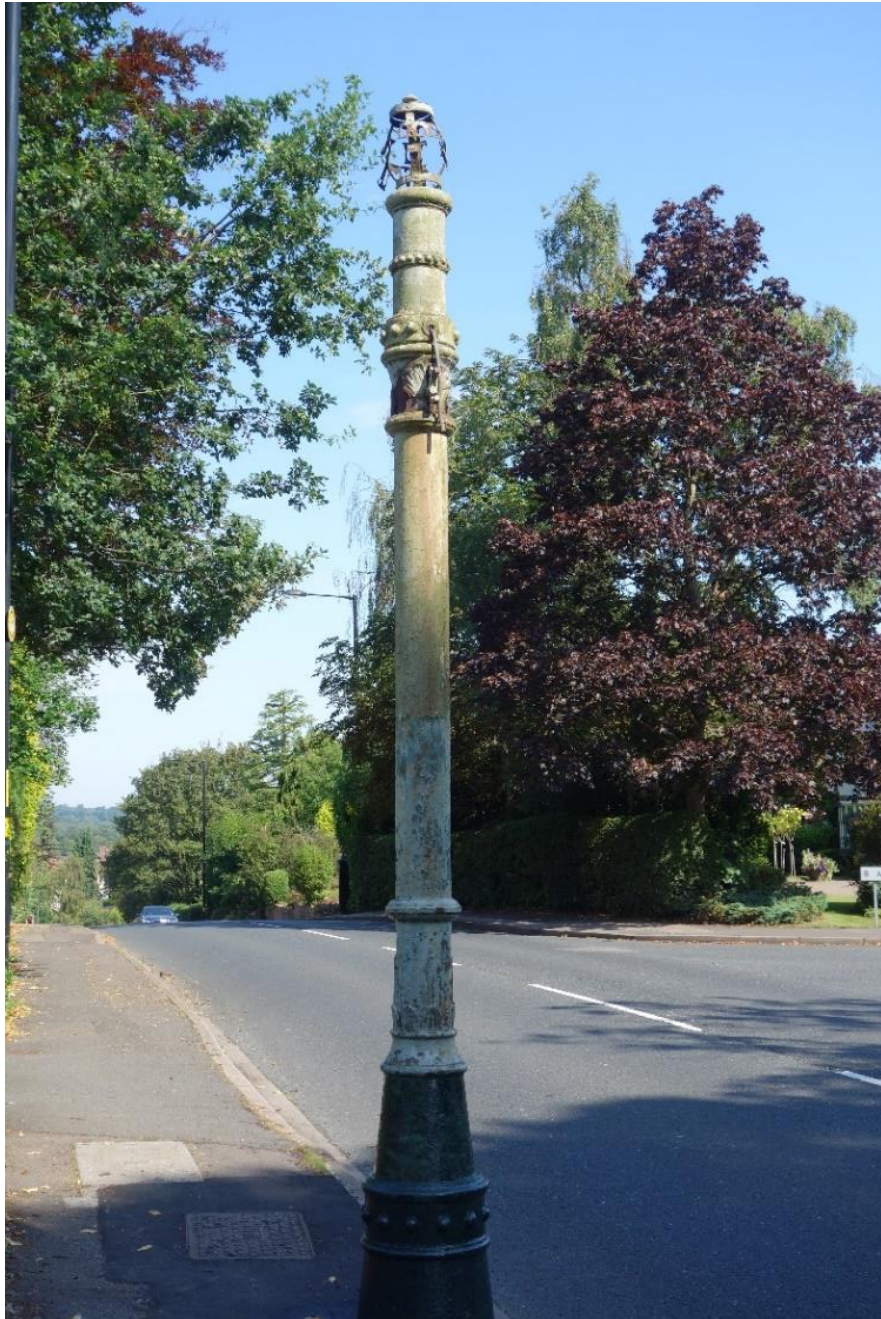
Photo 1 – The stench pipe in Somerville Road at O.S. G.R. SP1142 9530 looking northwards towards Monmouth Drive-Digby Road, Wyndley and Park Road. (Photo by author – 25.08.2019)
