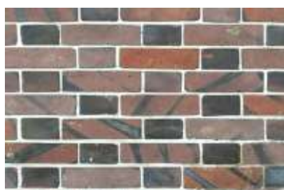
Fig. 1 An example of brickwork built in Flemish bond.
