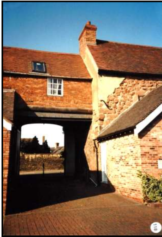
Fig. 6 The great archway, which led from the street into the yard, taken in 1995. Note the original exposed stonework behind the rendering.
