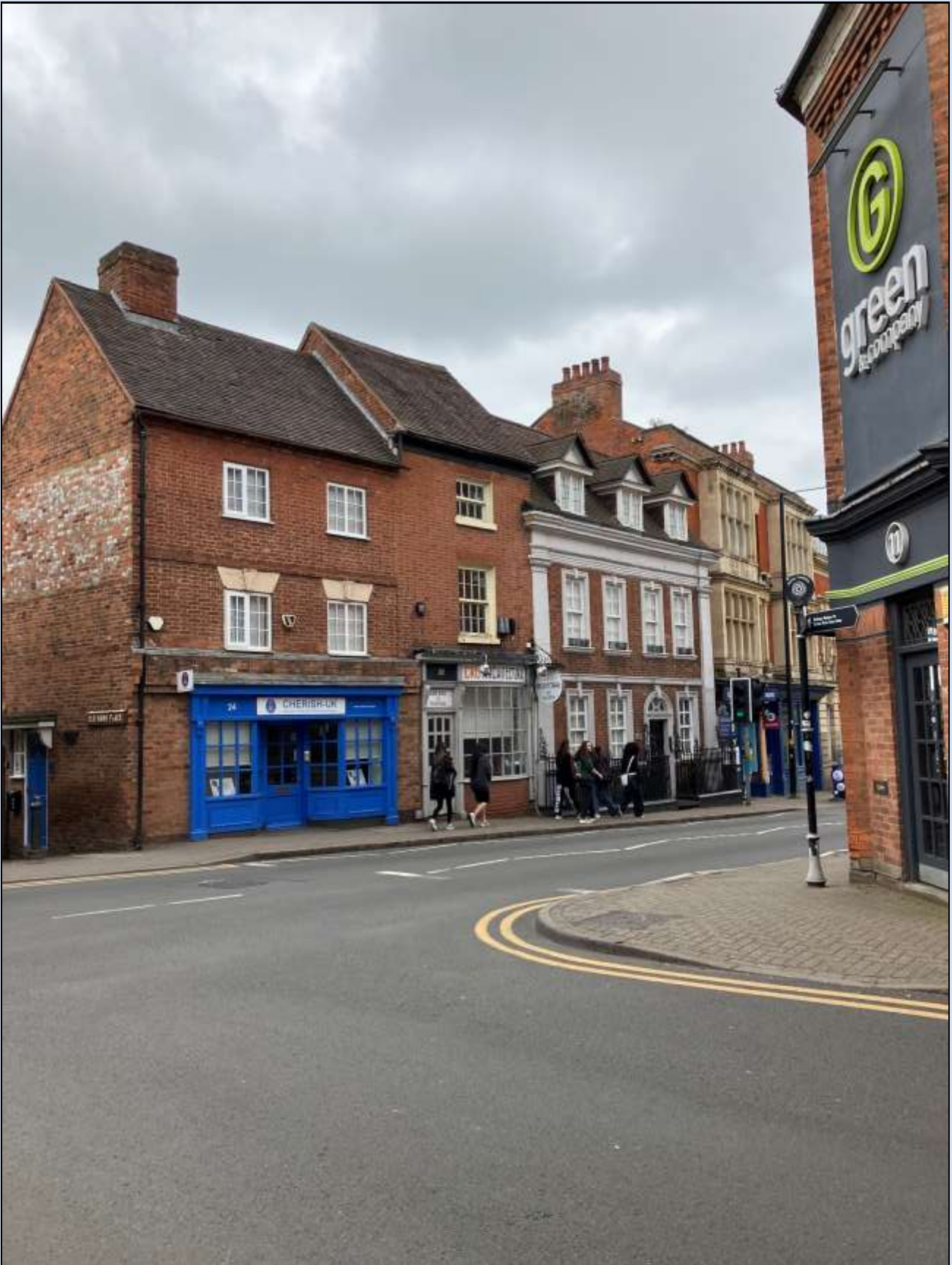
Author's photograph taken from Railway Road in 2025. Note the side of the converted White House, showing what I believe may have been the original chimney stack.
