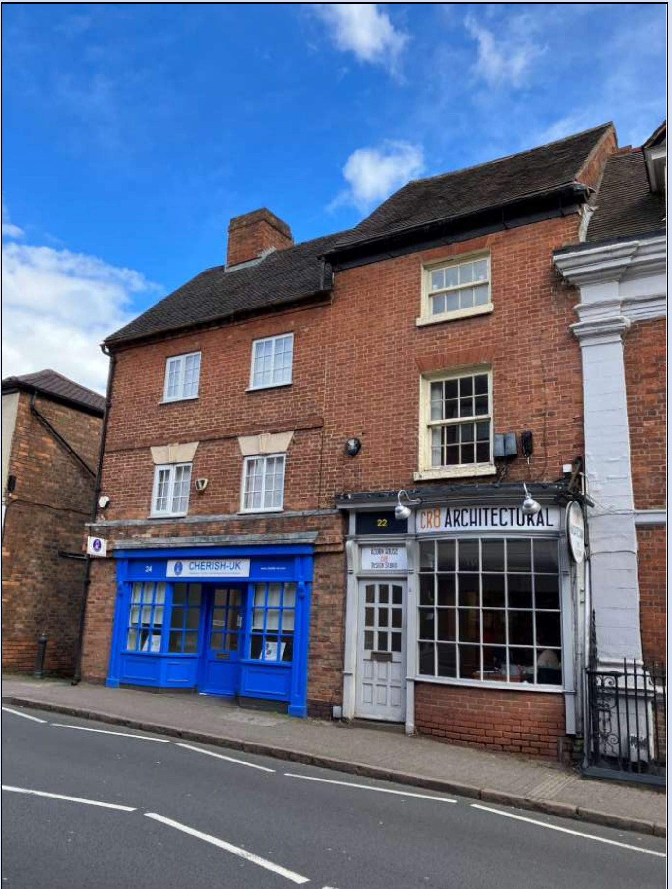
Author's photo taken in 2025 of 22 and 24 High Street. Note the two upstairs windows of No. 24 (See 1772 – photo of 24 High Street only has one upstairs window).
