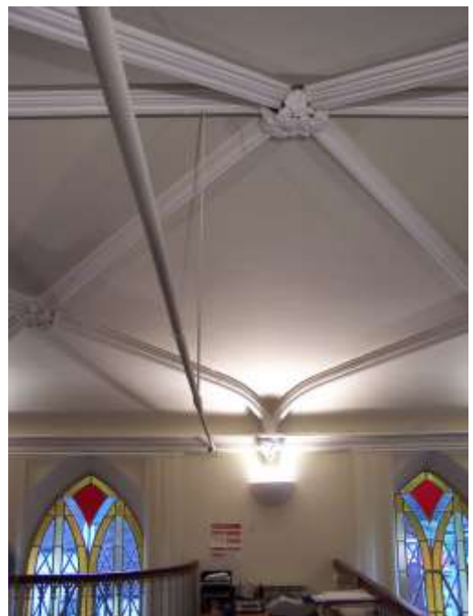
Fig 61 Roof showing cornice, roof ribs, tie beam and bosses
