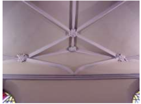
Fig 59 Roof showing cornice, roof ribs and bosses
