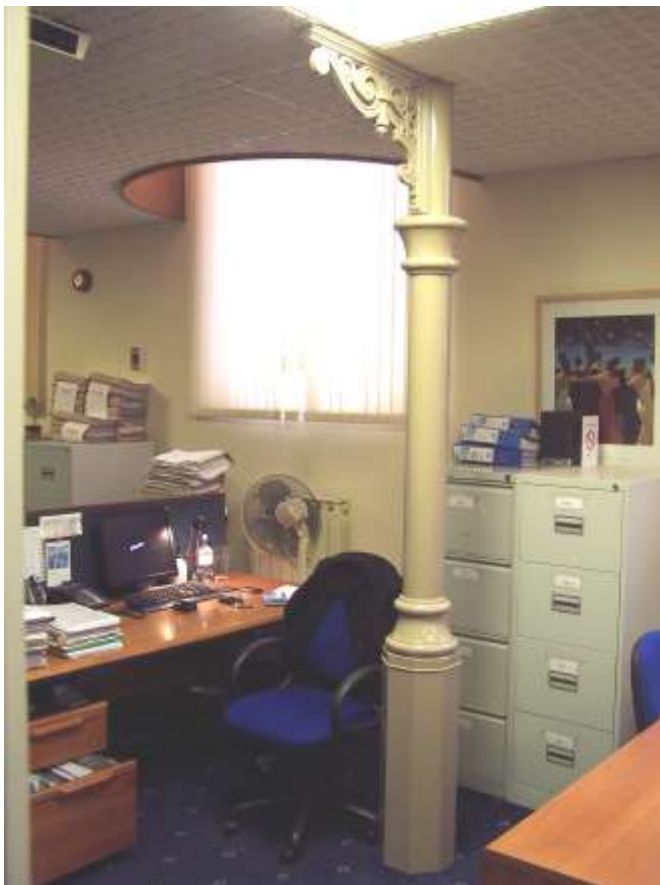
Fig 52 Ground Floor showing Victorian Pattern Cast Iron Columns and Beams
