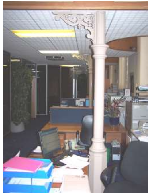
Fig 51 Ground Floor showing Victorian Pattern Cast Iron Columns and Beams
