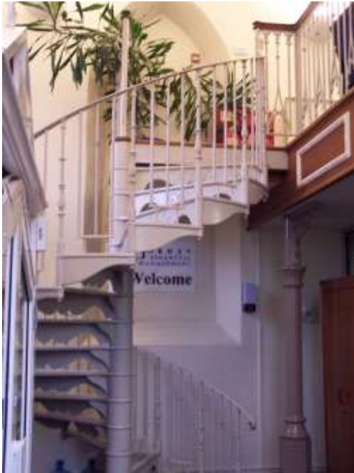
Fig 53 Victorian Pattern Cast Iron Spiral Stair, Balcony and Mezzanine Floor, 2008
