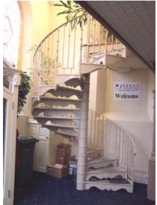
Fig 54 Victorian Pattern Cast Iron Spiral Stair, Balcony and Mezzanine Floor
