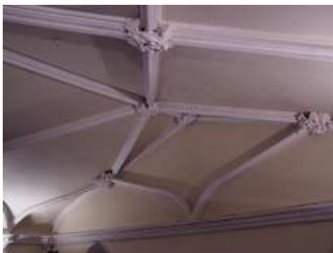
Fig 57 Roof showing cornice, roof ribs and bosses
