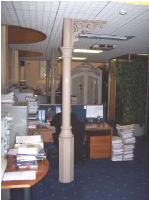
Fig 50 Ground Floor showing Victorian Pattern Cast Iron Columns and Beams, 2008
