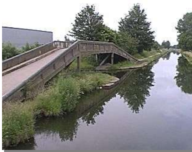
Wharf entrance to Sewage Works
