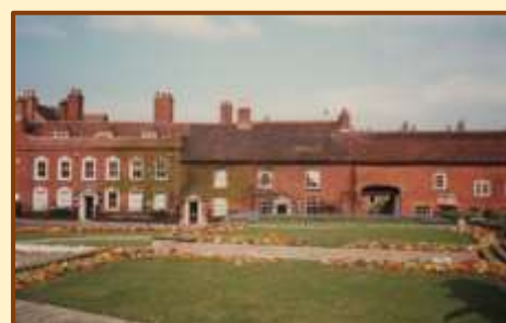
1-5 Coleshill Street, overlooking Vesey Gardens 1
