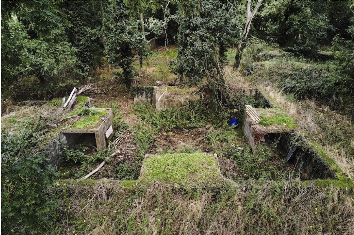
Figure 22. The Anti-aircraft site at Mautby, Norfolk. This is an identical design to the Streetly site, built at the same time. The four diametrically opposite ammunition shelters can be clearly be seen, a 3.7-inch gun would have sat on a circular base in the centre of each platform. The Command Post (below right) is exactly the same as that at Streetly.
