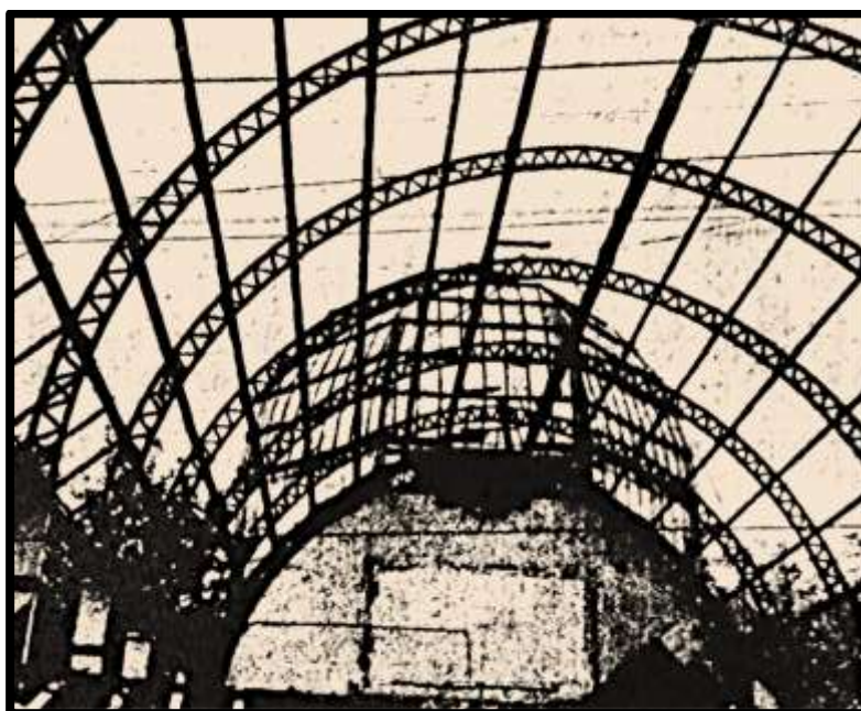
Fig. 44. A worm’s eye view of the interior of Sutton Coldfield’s old Crystal Palace , now in the course of demolition, with the glass panes removed, 1962.
