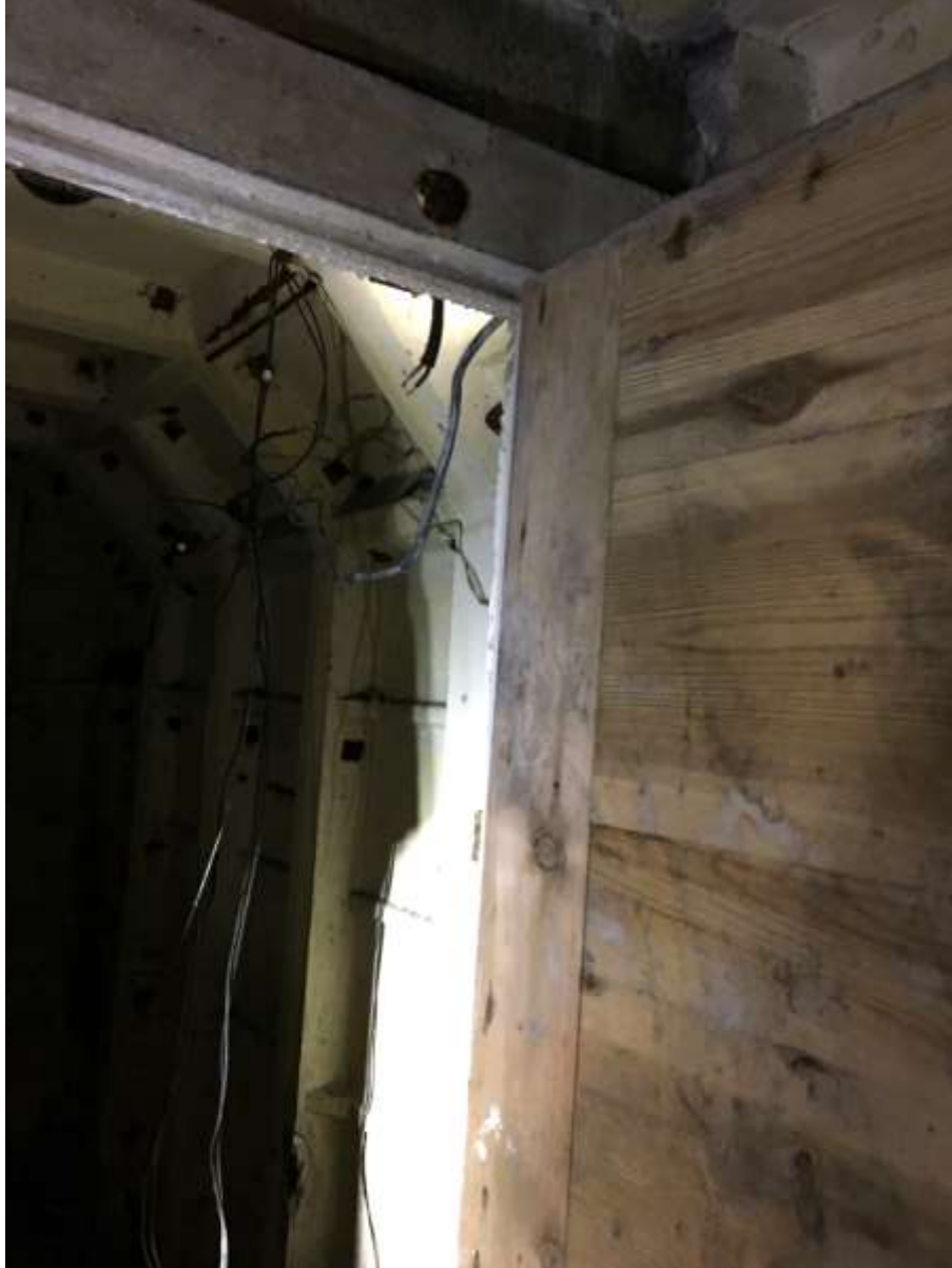
5. View of right hand side of shelter, showing its wooden door and electricity cables, which were connected to the house at the other end of the garden.
