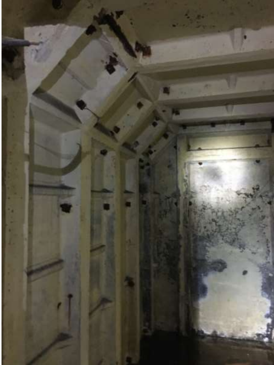
8. View of left hand side of shelter, showing 'Mansard ' shaped roof. The rear wall does not appear to be a door.
